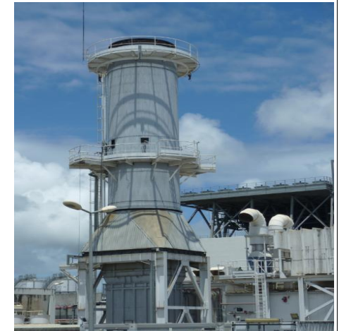
1x40 MWe Simple cycle GT in Guadeloupe (EDF)
